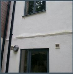
A schedule of works was agreed between SAS and the NHBC to replace the failed system with ProWall: SAS (Europe) Ltd's industry leading rendered rainscreen cladding system. SAS then set about appointing one of their trained approved applicators to first rectify issues the timber battening with and cavity space such as: Removing horizontal timbers at floor zones to allow for continuous ventilations and any further movement
